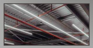
The lighting units together with the pre wired trunking reduce the time of installation and maintenance.
